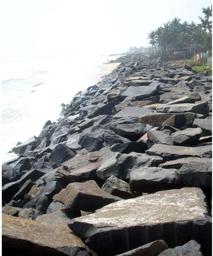
*Sea walls that have come along the coast of Pondicherry and Tamil Nadu have caused extensive erosion damaging property and infrastructure for many kilometres of the coast.*
