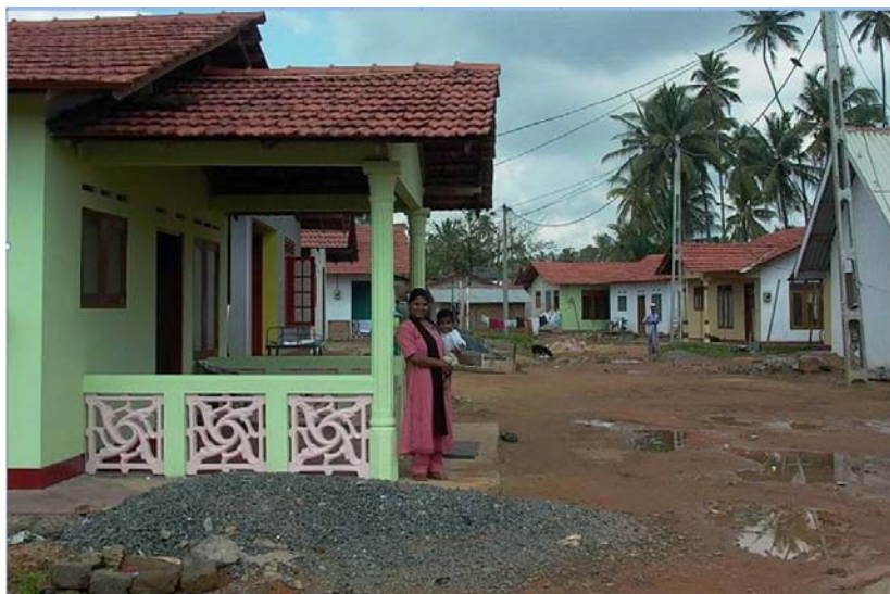
Completed People's Process Houses: Galle Sri Lanka.
